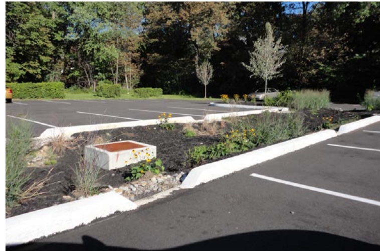
Curb cuts allow stormwater to flow into the central planting area in this parking lot in Cleveland Heights City Architecture
