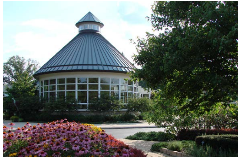
D.D. & Velma Davis Education & Visitor Center Mill Creek MetroParks
