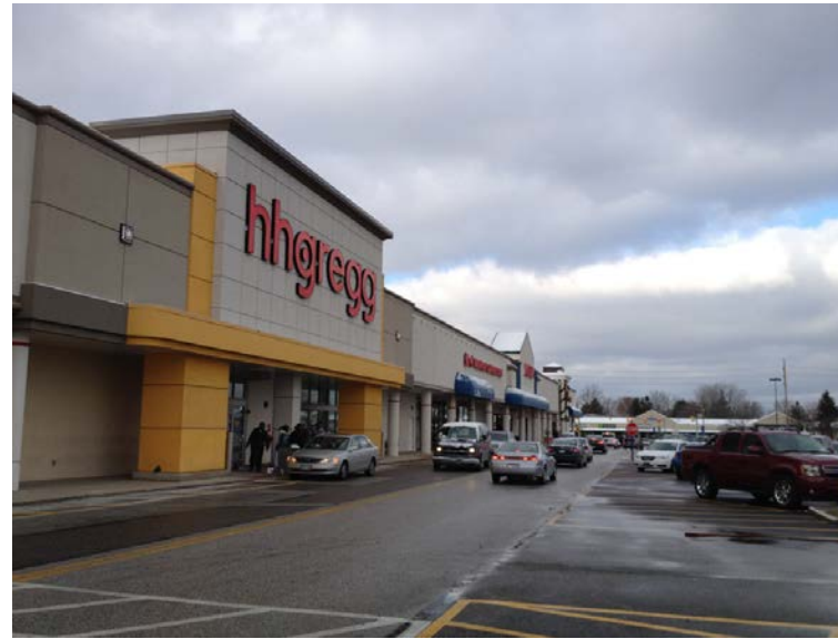
Golden Gate Strip Center City Architecture
