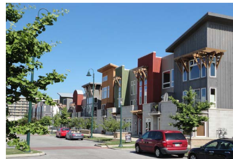
Battery Park Townhomes City Architecture
