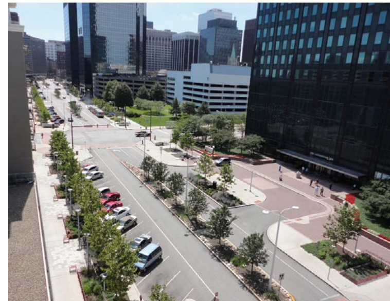
Example of a complete street in downtown Cleveland City Architecture
