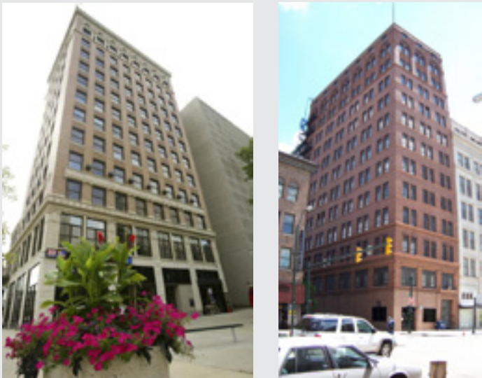
Realty Building and Wick Building City Architecture
